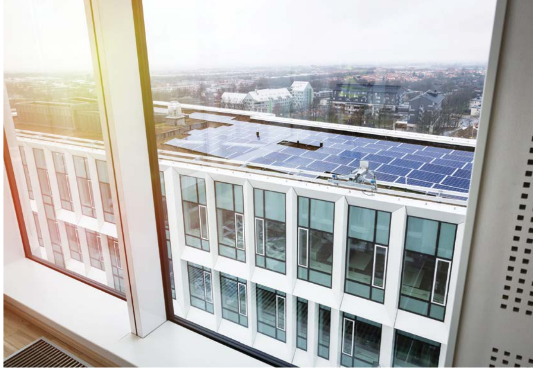
Solar panels on office roof.
