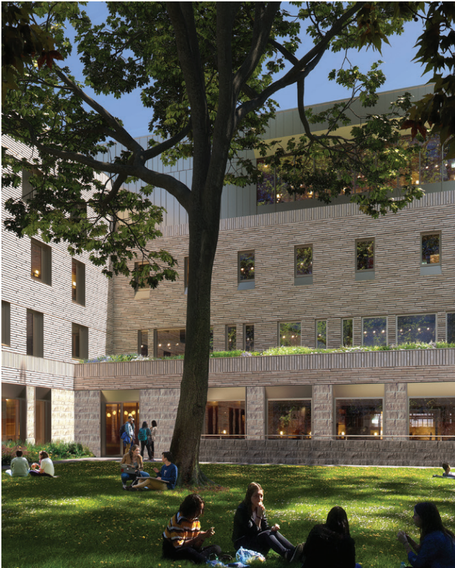
The Trinity College Lawson Centre for Sustainability and Acoustic Performance at the University of Toronto is dedicated to advancing sustainable design and optimizing acoustic excellence in a new mass timber, zero carbon, and LEED platinum multi-use building.
