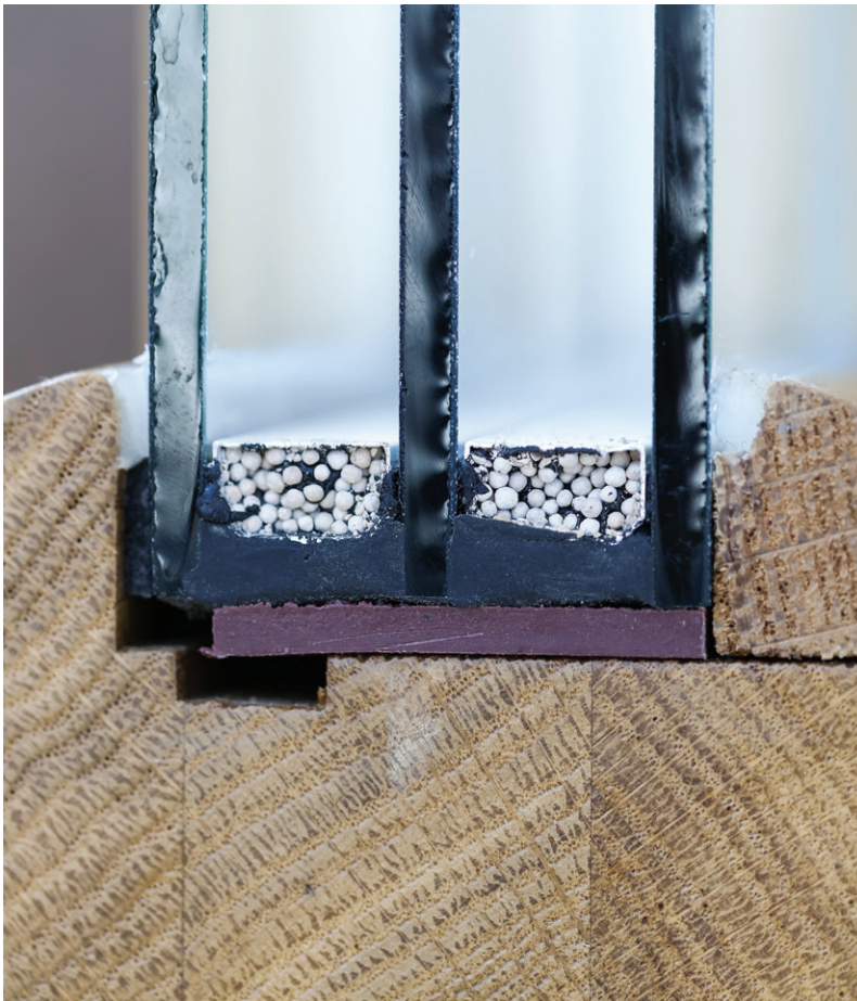
This cross section shows, in better detail, an example of a desiccant, spacer, and the sealant system.
