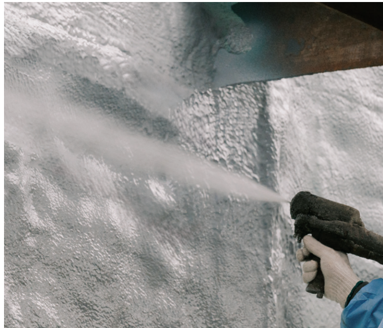
Contractor spraying the waterproofing coating over closed-cell sprayfoam.
