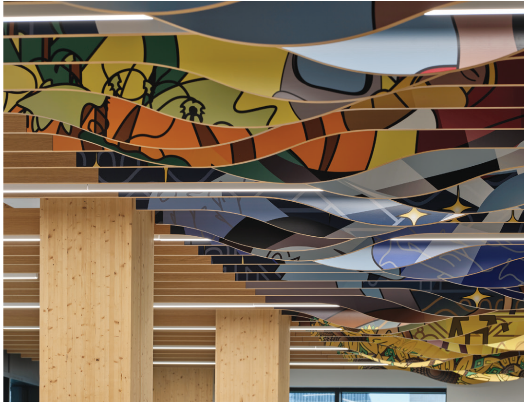
The ceiling treatment in Wisdom Hall at Centennial College's A-Building included custom wood baffles acting as absorptive panels to control acoustics. The acoustical baffles were incorporated into the story being told, so they did not interfere with the design.
