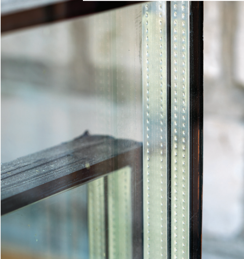
This shows a good representation of an edge seal in a finished unit.
