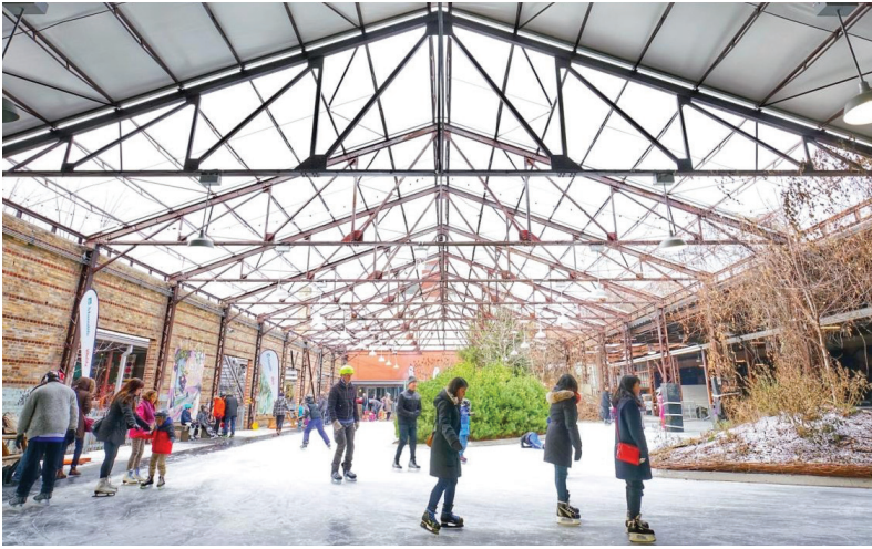
An example of adaptive reuse in action, the Evergreen Brick Works transforms a former industrial site into a vibrant community hub, featuring a seasonal skating rink that blends history with sustainability.
