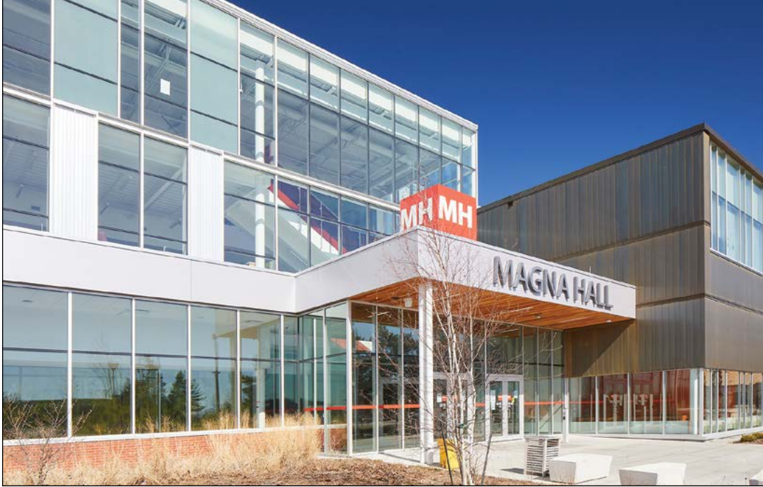
Seneca College's Magna Hall is designed with natural light, views, and energy efficiency. Aluminum-framed curtain wall with high thermal performance were specified to enclose the 21,554 m 2 (232,000 sf) academic and athletic building.
