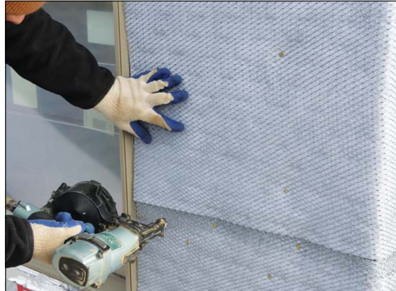
A factory-assembled mesh drainage plane and metal lath system offers faster installation and fewer wall penetrations than when installing the drainage plane and lath separately.
