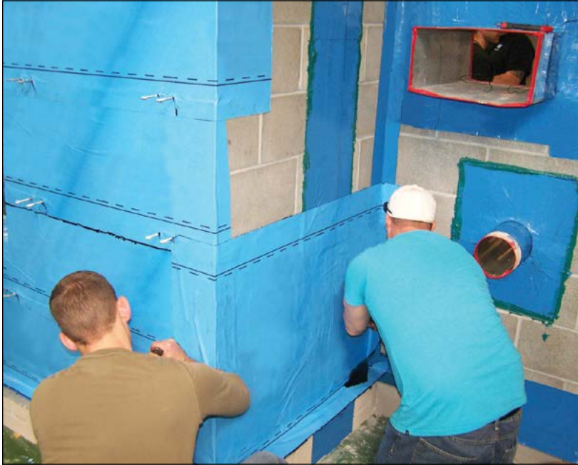
Air and weather barriers being installed on a façade comprised of concrete masonry units (CMUs).
