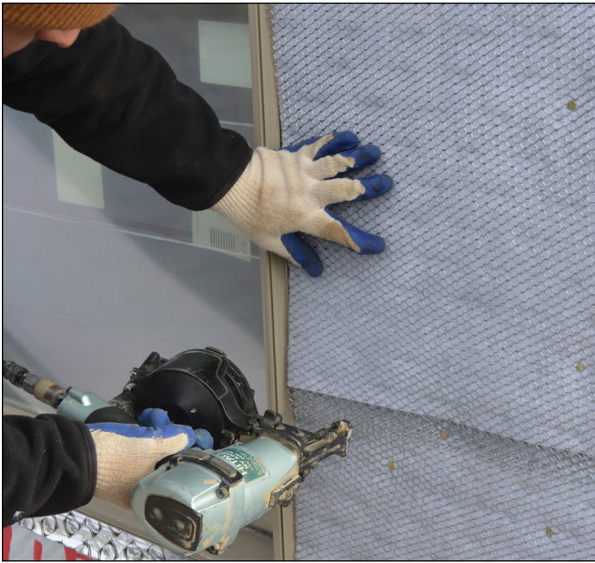
Factory-assembly metal lath and drainage plane systems install like regular lath.
