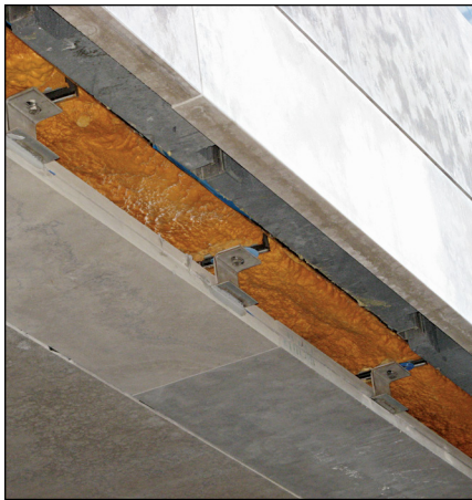
For natural stone, there are many new proprietary anchoring systems, some of which are back-anchored into the stone to allow for an open-joint rainscreen design. Examples include (from left to right): soffit anchor on strut, and two-piece anchors without or with di-electric separation.
