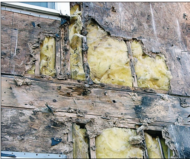
Mould and water damage resulting from a lack of drainage behind adhered masonry. One should note how the damage radiates from the bottom corner of the window, which is a typical location for leaks.
