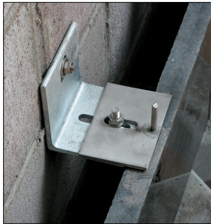
For natural stone, there are many new proprietary anchoring systems, some of which are back-anchored into the stone to allow for an open-joint rainscreen design. Examples include (from left to right): soffit anchor on strut, and two-piece anchors without or with di-electric separation.
