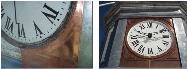
Copper recladding is underway. The image on the right shows the tower after recladding was complete.
