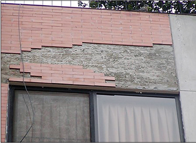
Thin-brick veneer popped off the substrate.
