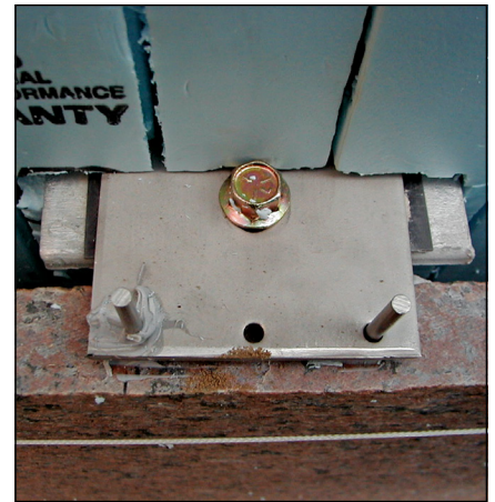
For natural stone, there are many new proprietary anchoring systems, some of which are back-anchored into the stone to allow for an open-joint rainscreen design. Examples include (from left to right): soffit anchor on strut, and two-piece anchors without or with di-electric separation.
